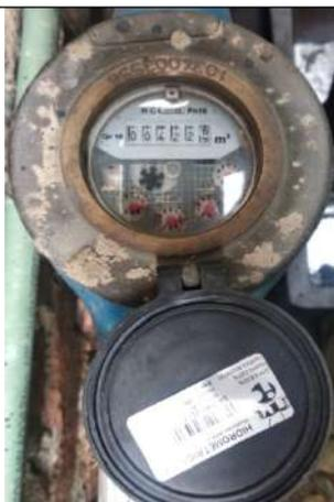
**Foto No. 7. Medidor No. 1034003556, lectura de 4226.5m<sup>3</sup>**
